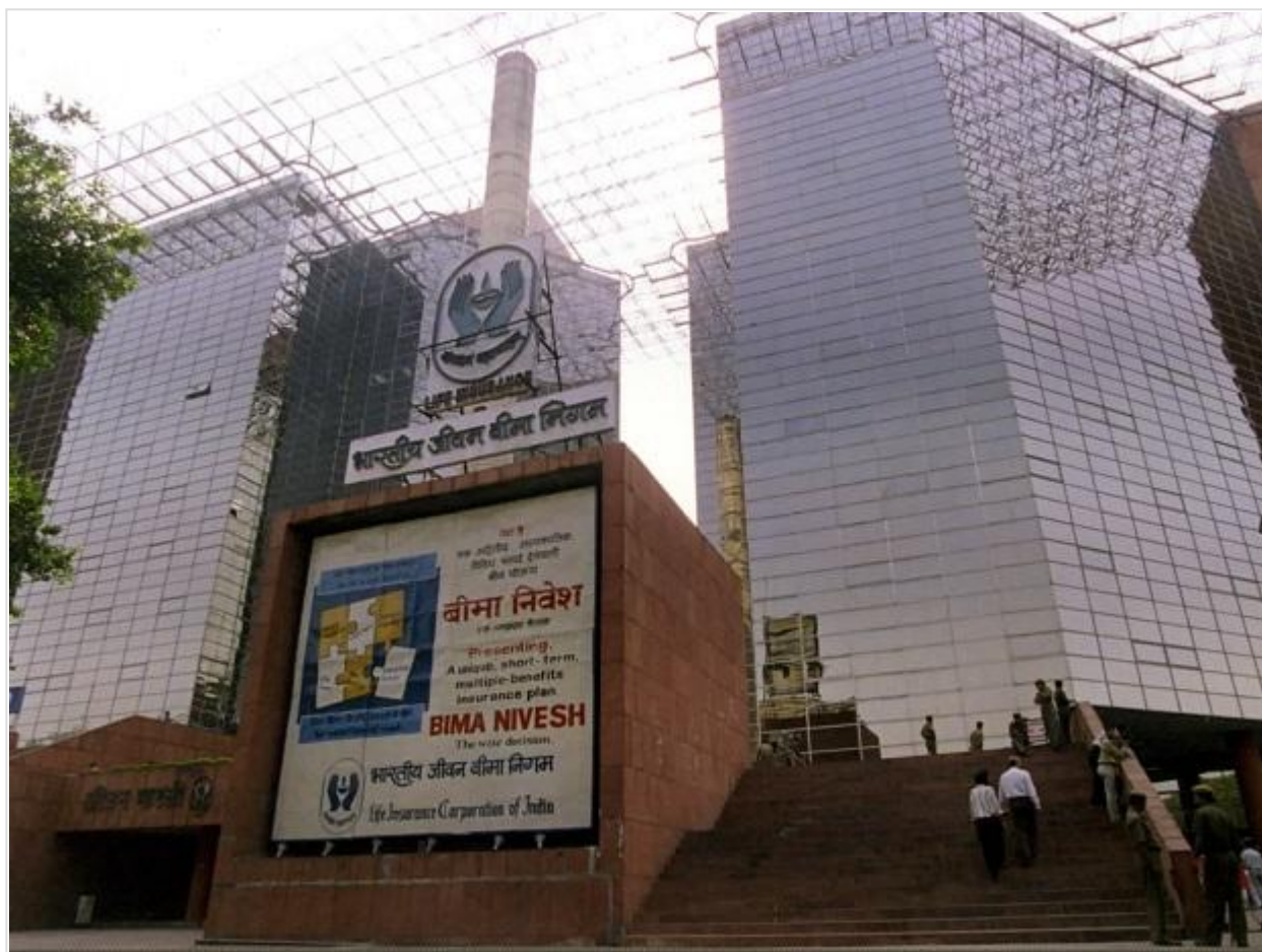
LIC building in Delhi
